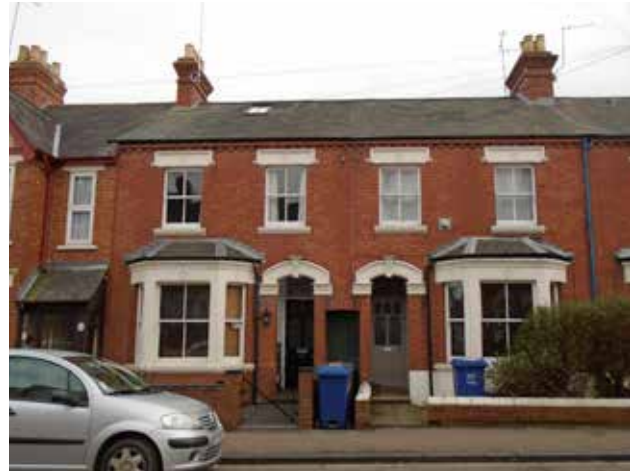
Queens Road 19th Century terrace housing
