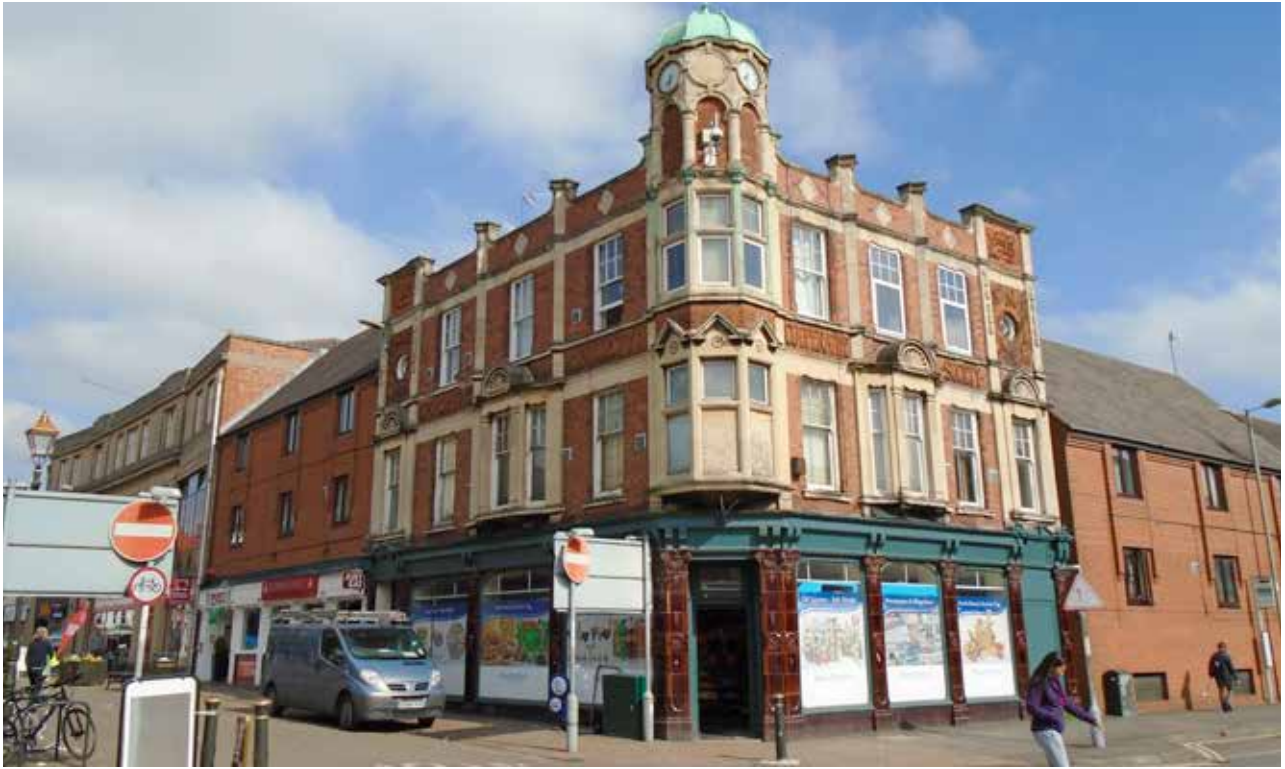
Banbury Co-operative building Broad Street
