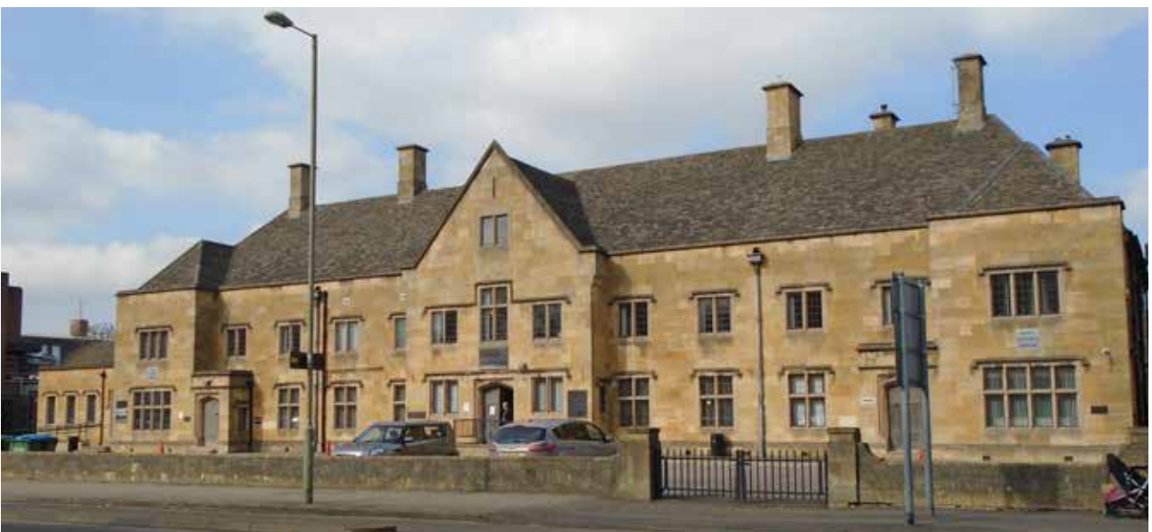
Banbury Court House
