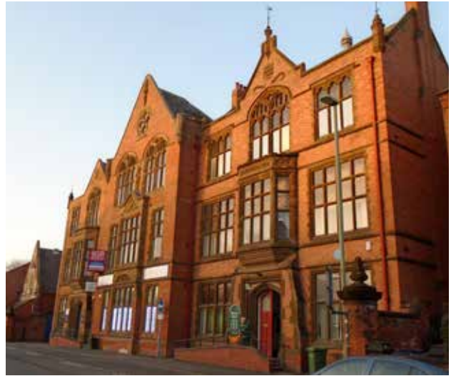
Public library Marlborough Road
