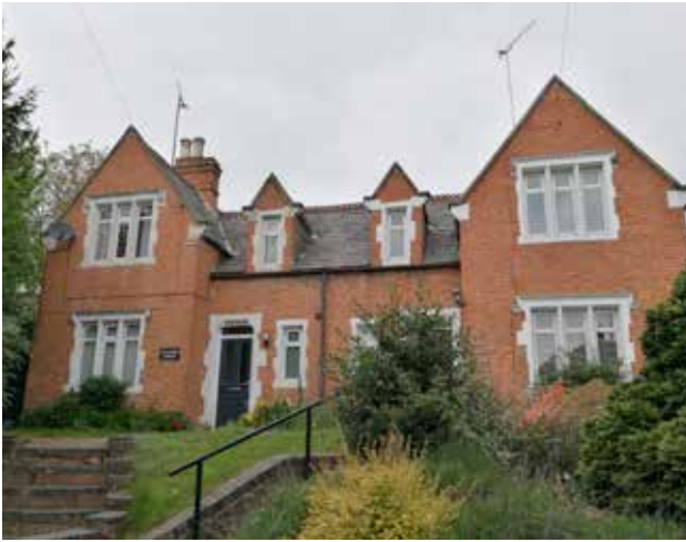
Union Master's House, Wartwick Road
